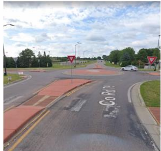
County Road 79 and Vierling Drive in Shakopee, MN
